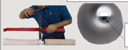
Edge of white cap should be in the center of the t-riser
